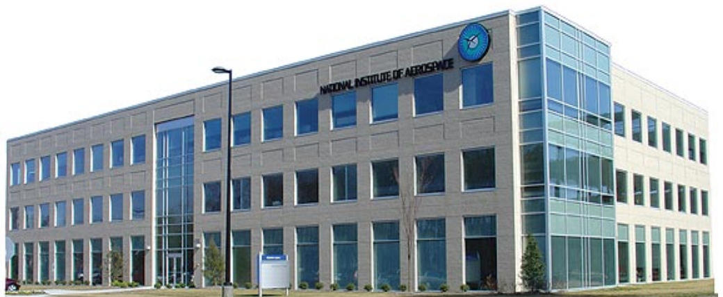
NIA Headquarters in Hampton, Virginia
